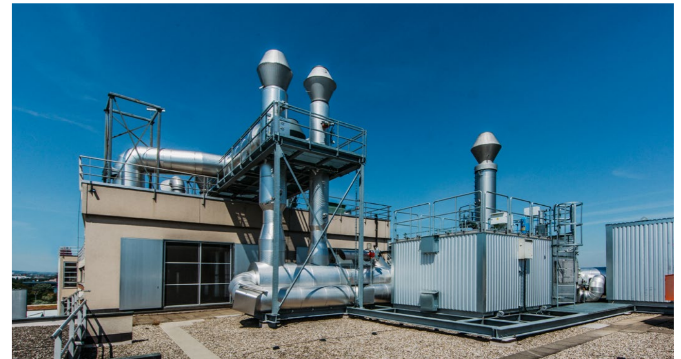
Electric exhaust air purification with 99.7 % VOC separation efficiency.
